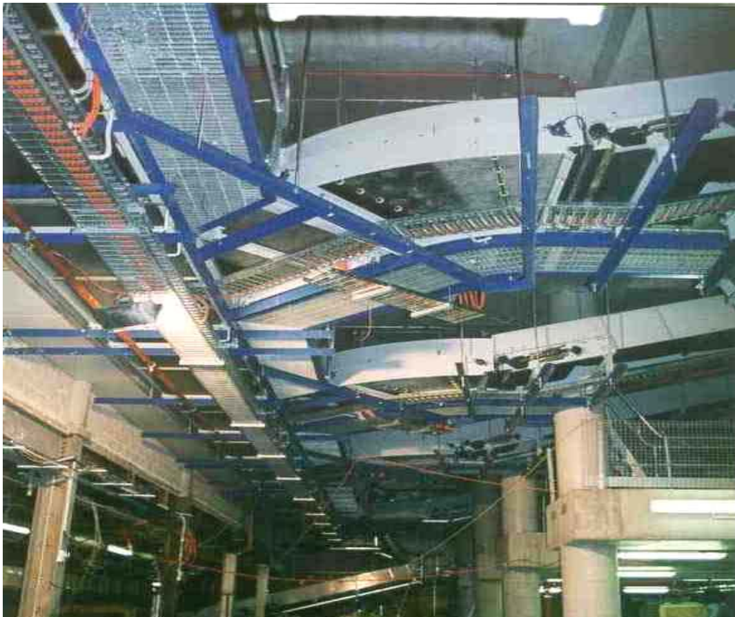
Underside of power curves, catwalk and 45 degree merges
